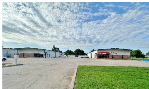
59th Street Warehouses 3200-3208 S.W. 59th Street-OKC 22,640 SF
