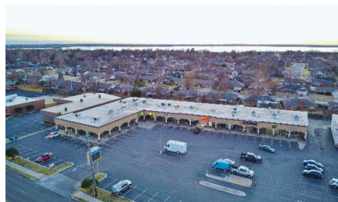
Village Park South 10407 N. May Avenue-OKC 22,573 SF
